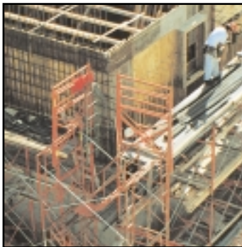
1.2.1.2 Tower Shaft Structural
